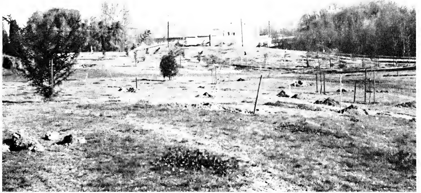
Holes being dug for the trees. Photo: J.A. Witt
